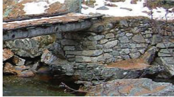
Dry set masonry supports a rustic log bridge, where it provides a well - drained support for the log (which will increase its service life)
